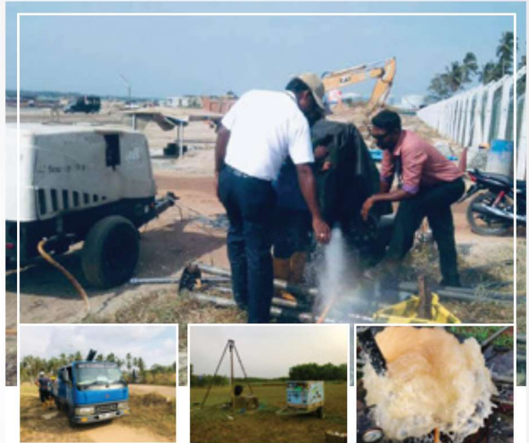
Airport, Katunayake 15 Deep Tube Well Development project
