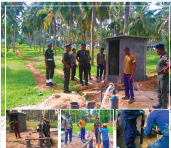
Boyagane Army camp Deep well water project @ Vijayabahu Infantry regiment
