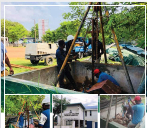
Thurstan College Deep Tube Well flushing and Submersible pump service
